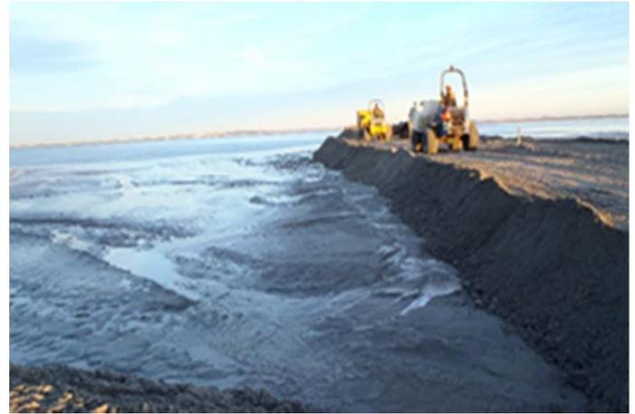
Fig. 3. Trial embankment during formation.
